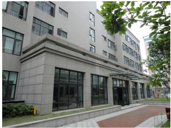
厂房/Plant Building
