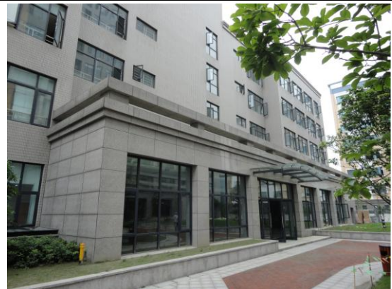
厂房/Plant Building
