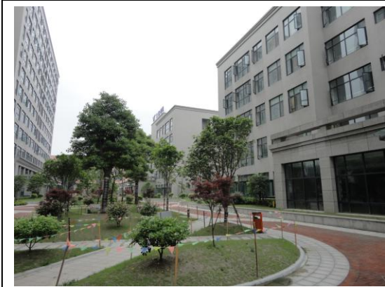
金润高科园区/Jin Run High Tech Park
